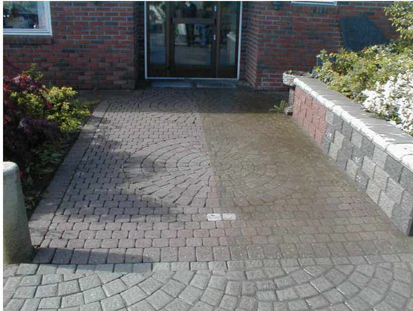
Roof tile & sidewalk cleaning & washing
